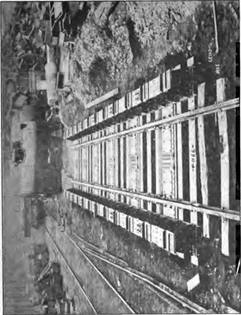
FIRING PLATFORM FOR THE 12-INCH, 3-CALIBER AMERICAN GUN MOUNT.
